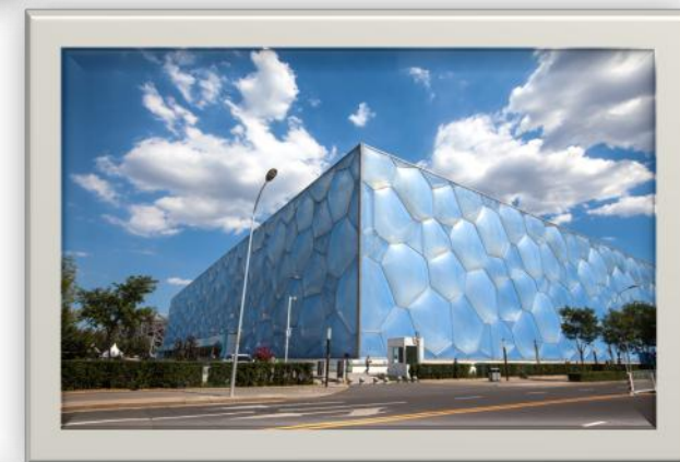
The Water Cube (National Aquatics Center) 2008 Summer Olympics
